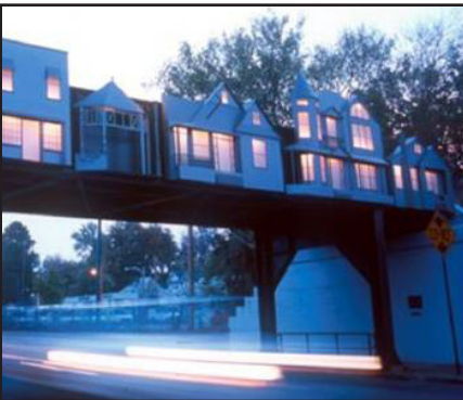
Incorporating public art into infrastructure and the built environment can be an engaging way to stimulate activity, conversation and general interest in the area.
