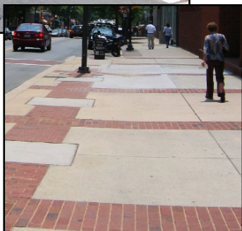
Different pavement treatments such as applied brick rendering (above) and combining brick and concrete help to identify pedestrian crossings and distinguish between pedestrian and motorist zones.
