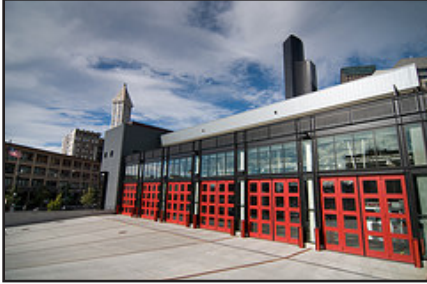
This fire station takes advantage of its urban location in terms of siting and design with contemporary features.
