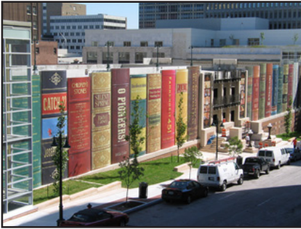
This parking garage was screened with a facade composed of book bindings to articulate the sidewalk, add visual interest and incorporate public art.
