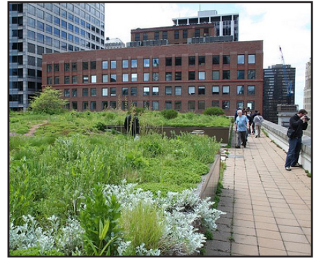
The vegetated roof on this structure limits its impact on heat islands, reduces its energy usage for heating and cooling and provides for an alternative green space within the urban environment.
