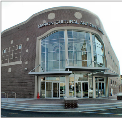
The entrance to this cultural center is directly accessible from the street with distinct features that acknowledge the principle entrance such as the use of glass, multi-level canopies, and signage.
