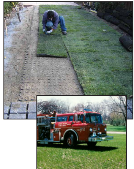
Porous paving systems allow for infiltration, can reduce stormwater runoff and provide open, green space while providing alternatives for parking paving systems.
