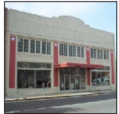
The entrance to this building uses a canopy structure and an accented parapet to give an unassuming entrance more prominence.
