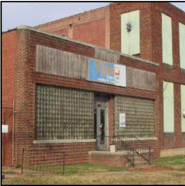
The glass block on this industrial building helps to define its historic context as well as its individuality.
