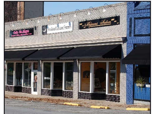
This strip shopping center employs individual signage and uses individual awnings for each business.
