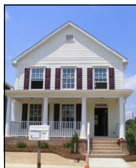
Phase II Construction
