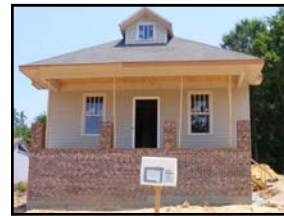
New Single Family Home Construction by Self-Help
