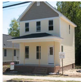
New single-family construction
