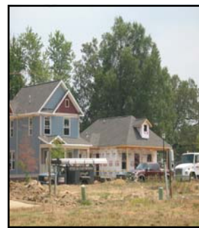
Phase II Construction
