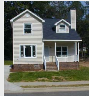
A completed house in The Village at Arlington Park.
