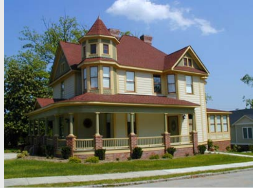
The rehabilitation of 400 Gorrell Street was completed this fiscal year. All of the historic houses in Southside are now under contract or in rehabilitation.
