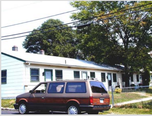
The four apartment complex structures on Gillespie Street will be demolished and re-planned in the next fiscal year.
