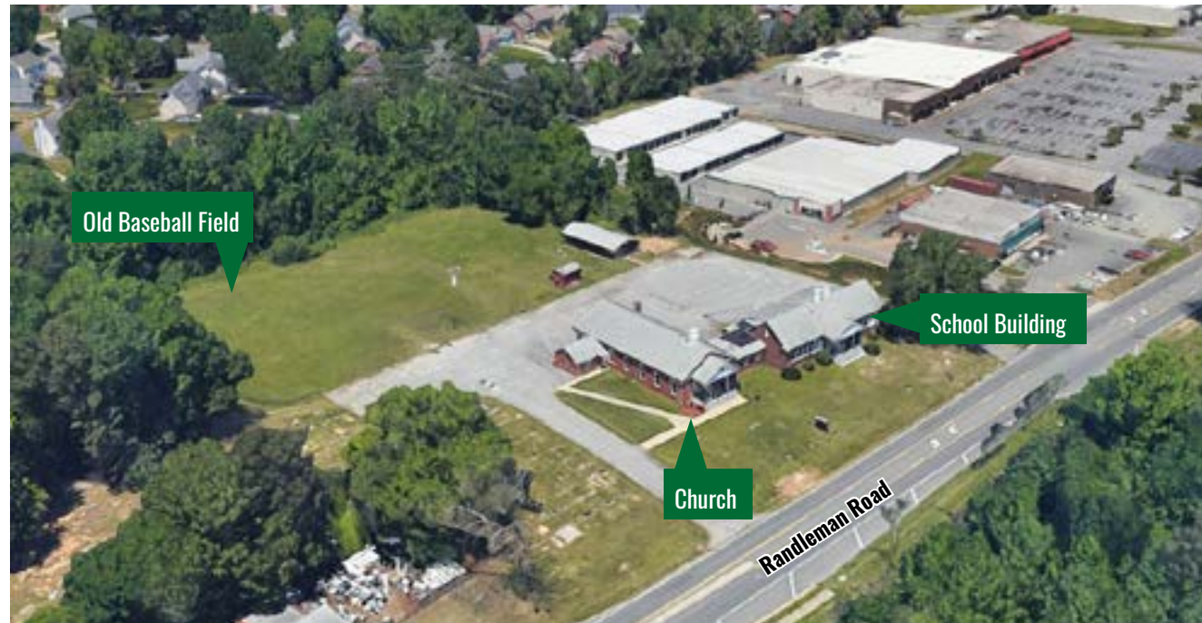
New Goshen United Methodist Church Site. Source: Google Earth
