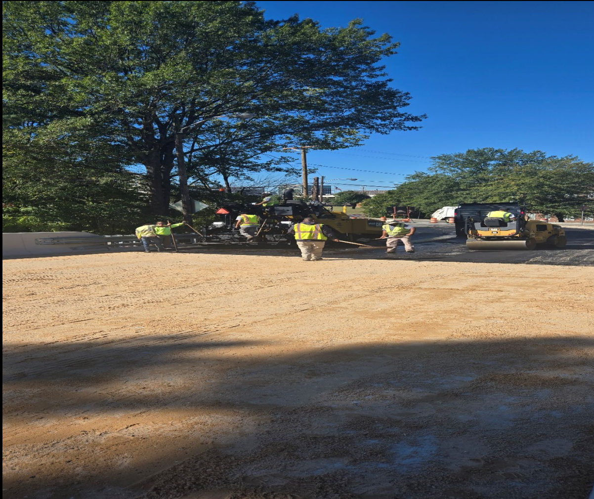
Murrow Boulevard Bridge over Church Street
