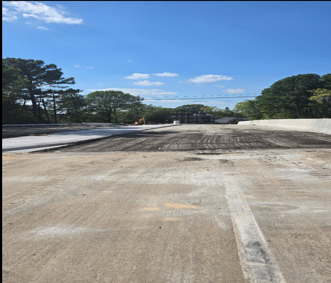
Murrow Boulevard Bridge over Church Street
