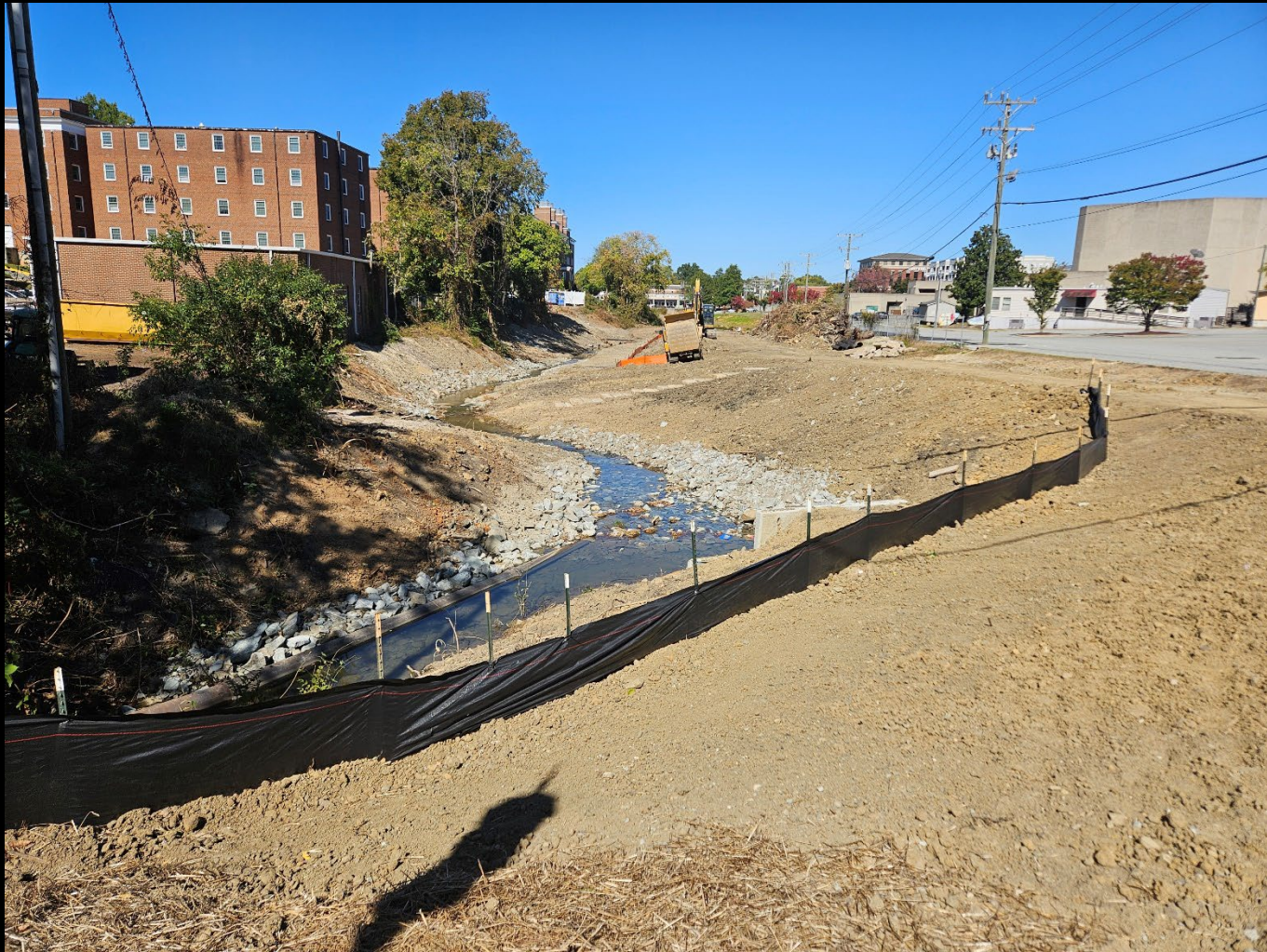
Downtown Greenway – Stream Restoration near McGee Street
