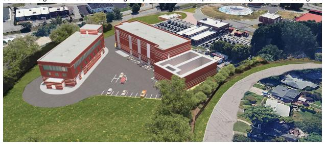
Regarding building setback, it should be noted that existing plant structures are currently within 15 feet of the fence. As noted in City Council Resolutions, this new property was purchased to provide space for additional treatment and capacity as the City's needs grow and change. Based on this need, new development at the site will be set back at least the minimum 45-feet from the property line to allow the City flexibility in future development.
