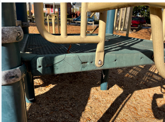
Playground Conditions at Douglas Park
