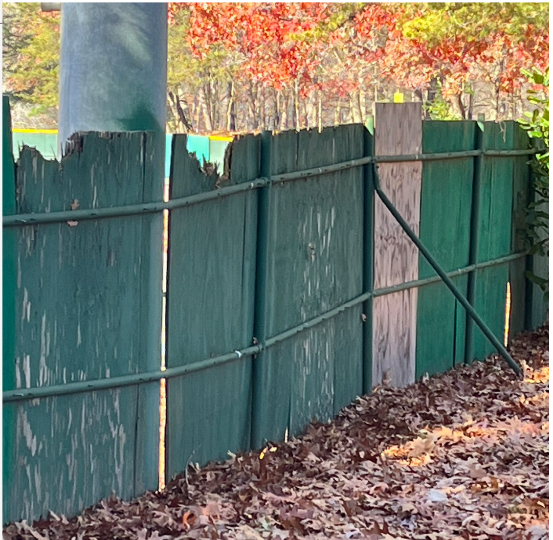
Stoner-White Stadium Fence
