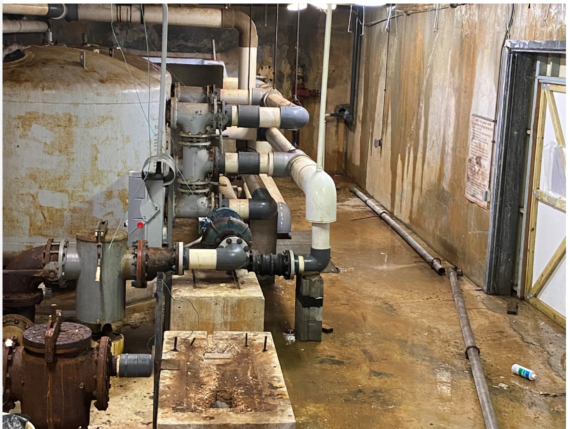
Pump Room Condition at Lindley Pool
