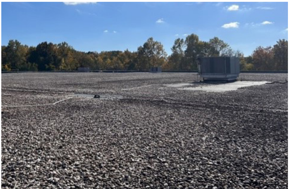
Existing Roof at the Greensboro Sportsplex
