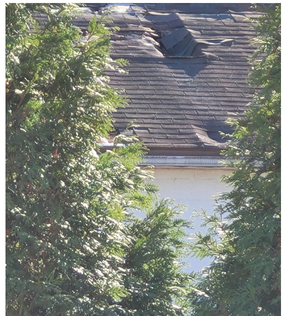
Gillespie Maintenance Building Roof
