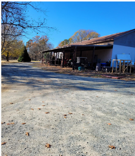
Gillespie Maintenance Building
