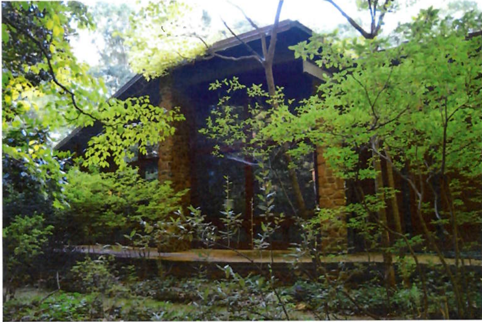
Façade, view north.
