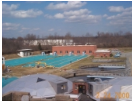
North Buffalo Plant (located off of White Street)
