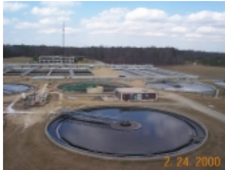
T. Z. Osborne Plant (located off of Huffine Mill Road)
