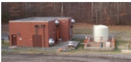
Rock Creek Pump Station
