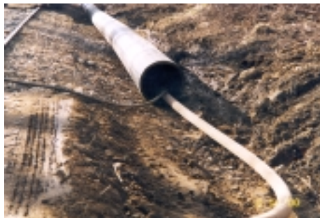
Sewer Pipe Slip Lining (refurbishing old lines)
