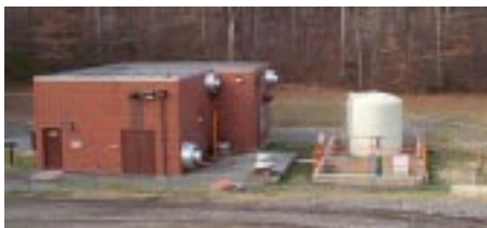
Rock Creek Pump Station
