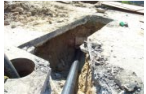
Sewer Line Rehabilitation
