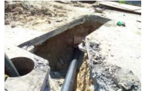
Sewer Line Rehabilitation
