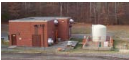
Rock Creek Pump Station
