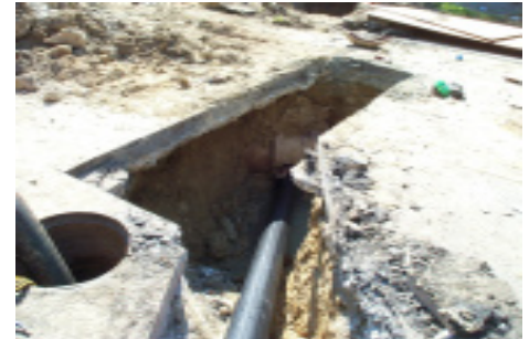
Sewer Line Rehabilitation
