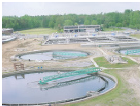
T. Z. Osborne Plant (located off of Huffine Mill Road)
