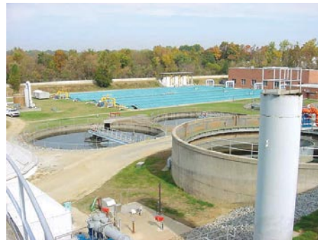
North Buffalo Plant (located off of White Street)
