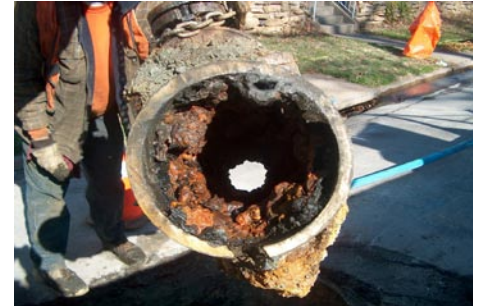
Sewer Line Rehabilitation
