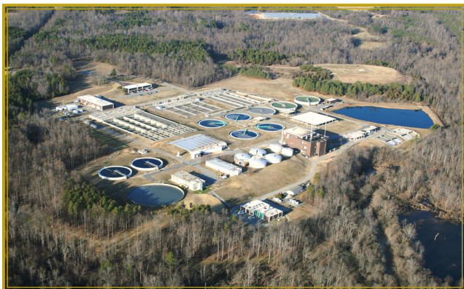
Aerial photo of T.Z. Osborne Plant
