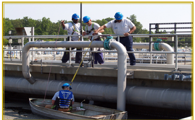
Facility maintenance by wastewater staff
