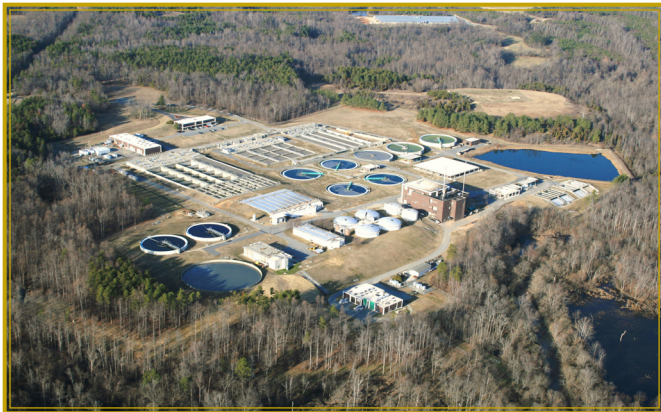
Aerial photo of T.Z. Osborne Wastewater Plant
