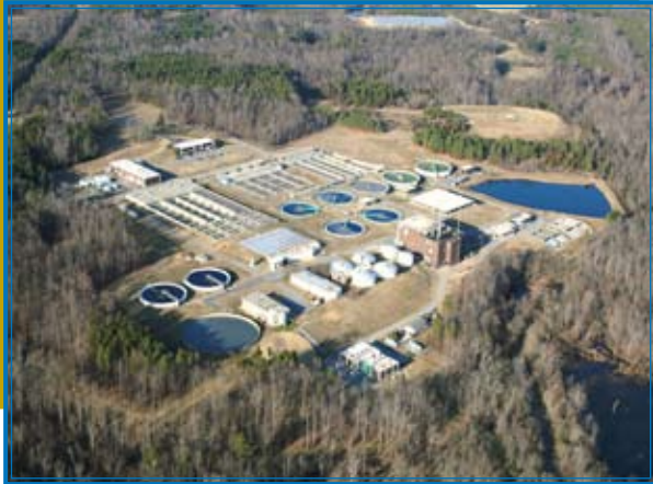
Aerial photo of T.Z. Osborne Wastewater Plant
