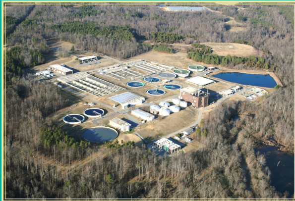
Aerial photo of T. Z. Osborne Wastewater Plant
