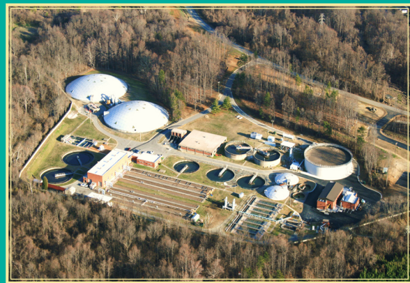
Aerial photo of North Buffalo Wastewater Plant
