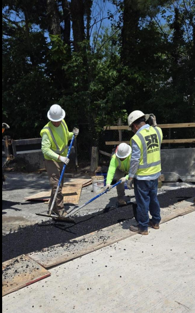
Murrow Boulevard Bridge over Church Street
