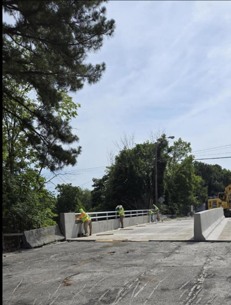
Murrow Boulevard Bridge over Church Street
