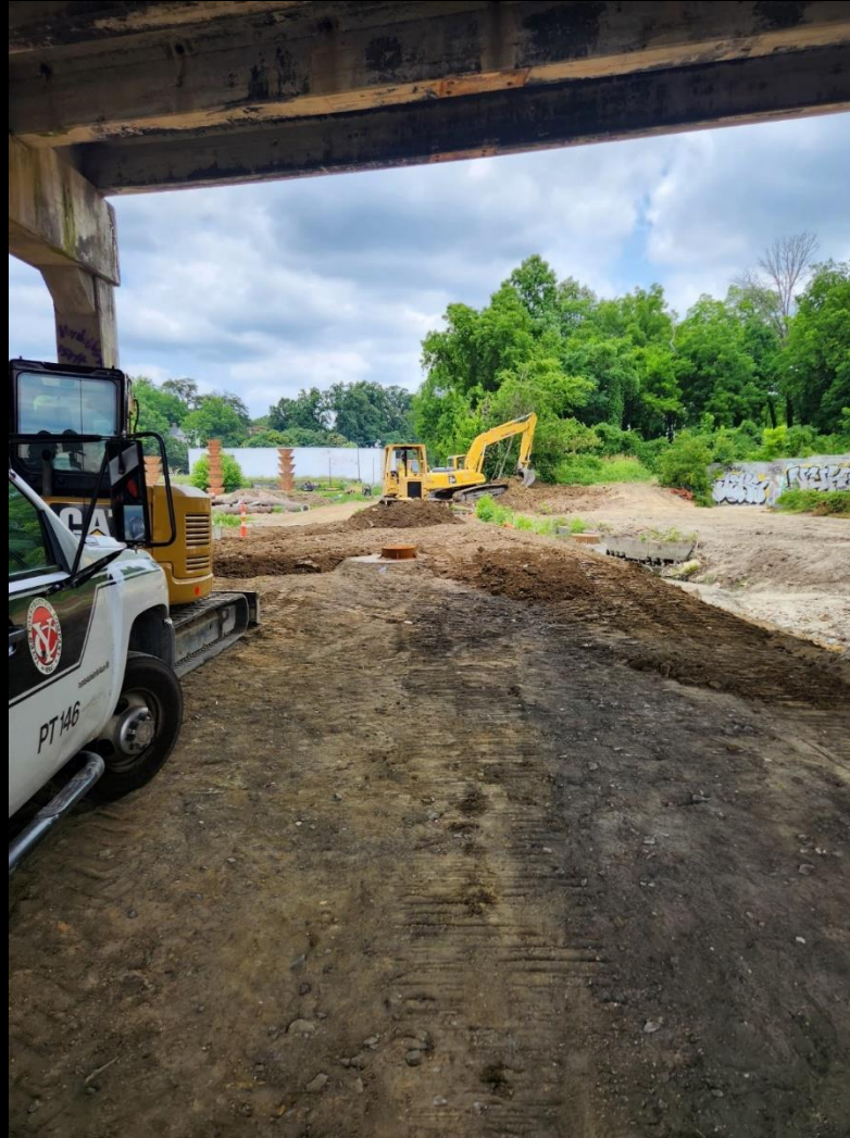
Downtown Greenway – Utility Work under Friendly
