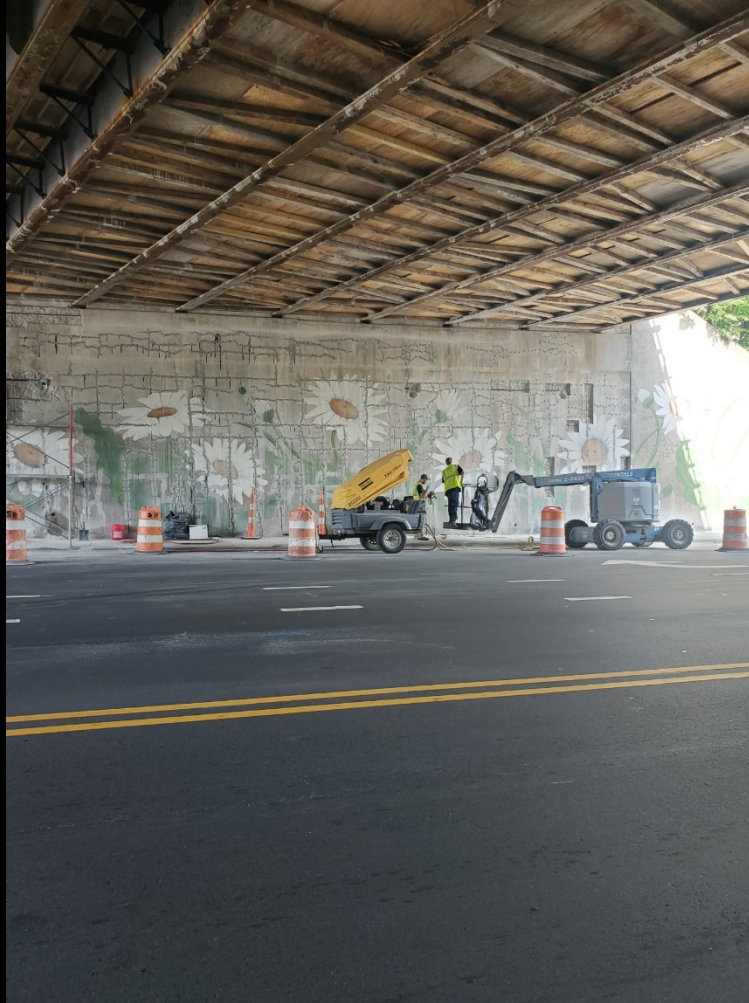
Murrow Boulevard Bridge over Church Street
