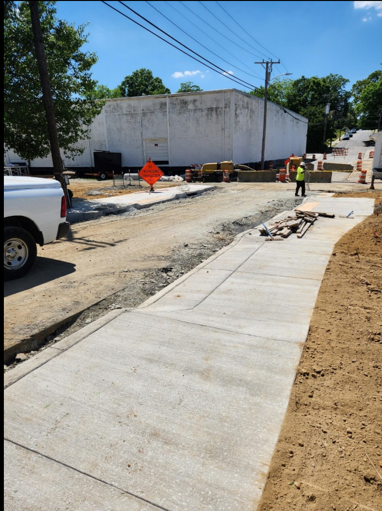
Downtown Greenway – Guilford Avenue Improvements
