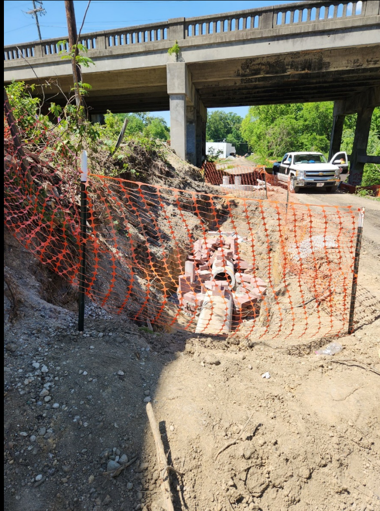
Downtown Greenway – Drainage under Friendly Avenue
