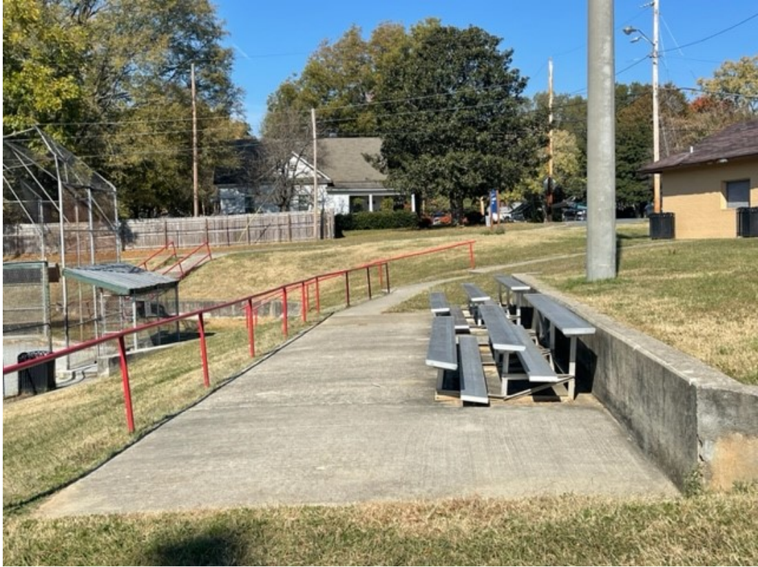
Existing Conditions at Field
