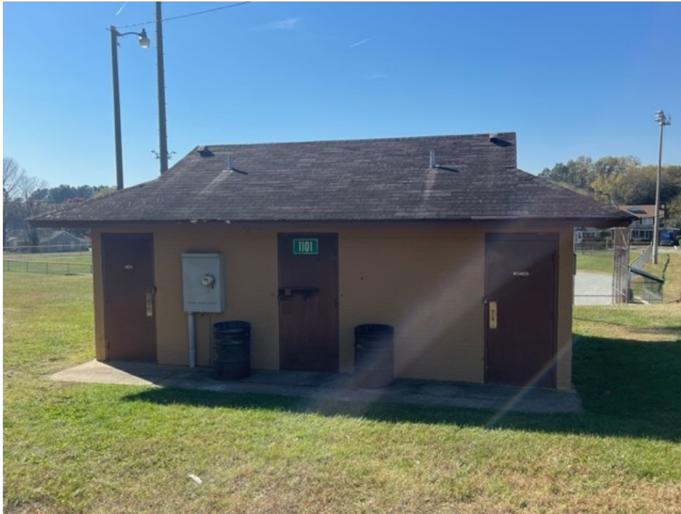
Existing Restroom Building
