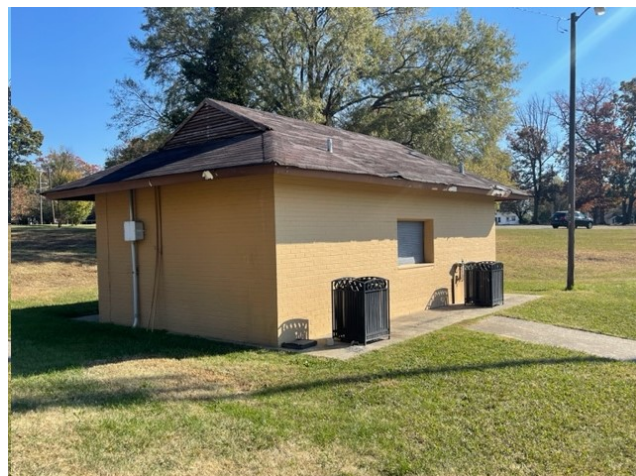
Existing Bathrooms and Snack Bar
