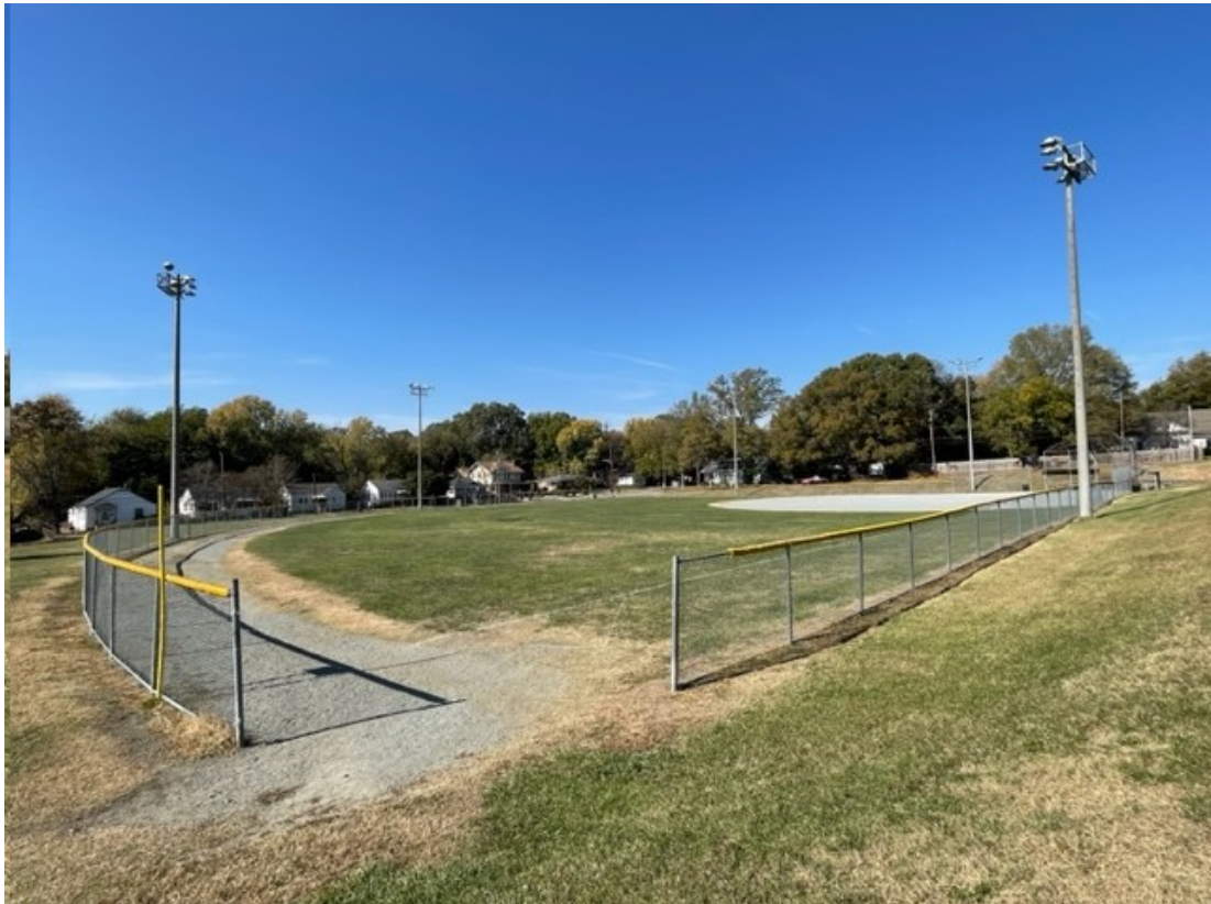
Existing Conditions at Field
