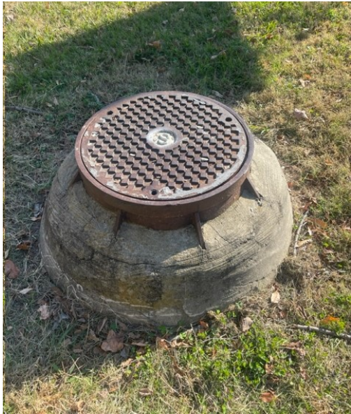
Sanitary Sewer Manhole
