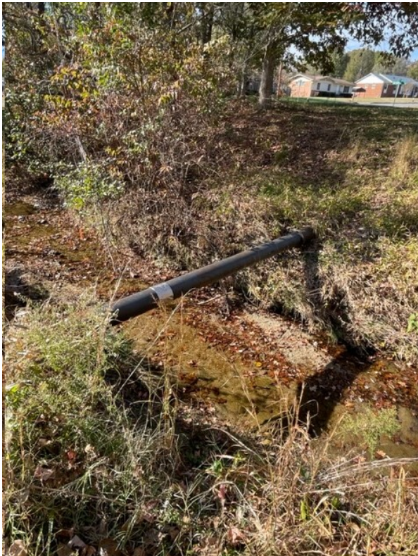
Aerial Sanitary Sewer Crossing
