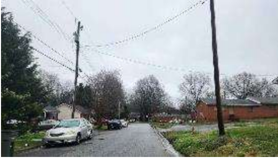
Looking East on John Dimrey Drive
