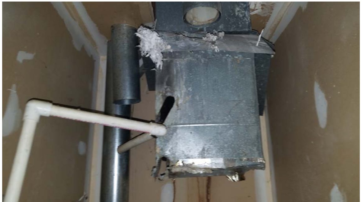
Example of attic insulation throughout each unit.
