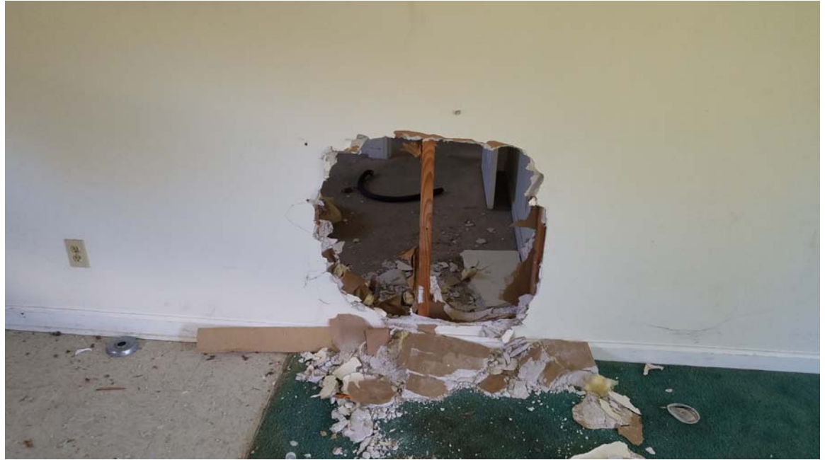
Example of drywall and patch throughout each unit.
