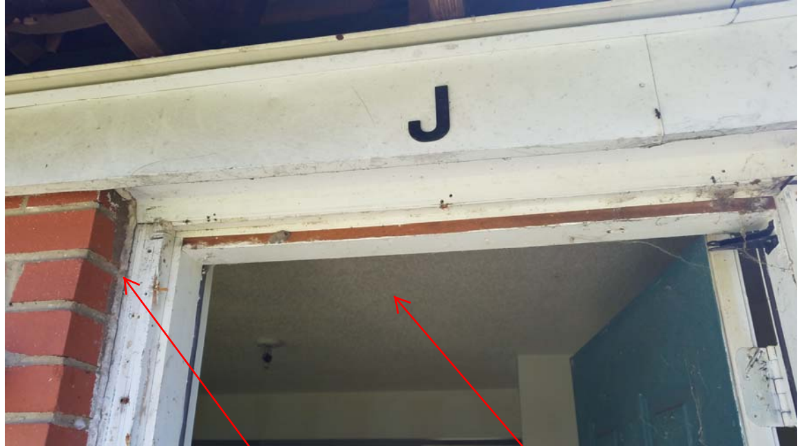
Example of exterior caulking and interior ceiling texture.
