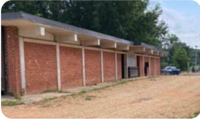
⬆ Exterior of the pool house at Peeler Recreation Center
