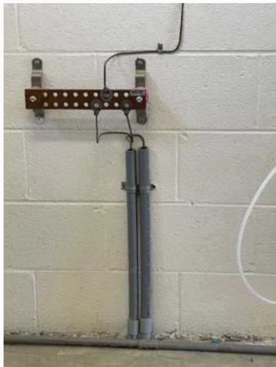
Figure E6 – Bonding Conductors
