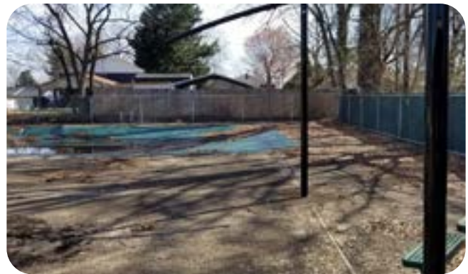
Deck covered in leaves and a deteriorating pool cover
