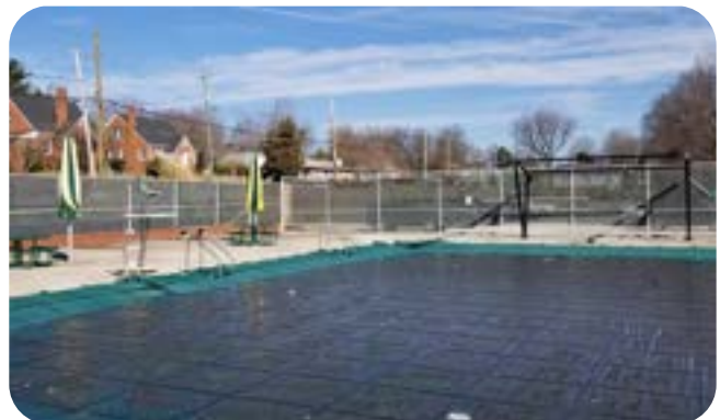
▲ Pool deck, furnishings, and winterized shade structure
