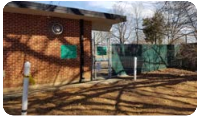
Secondary entry to pool area from parking lot
