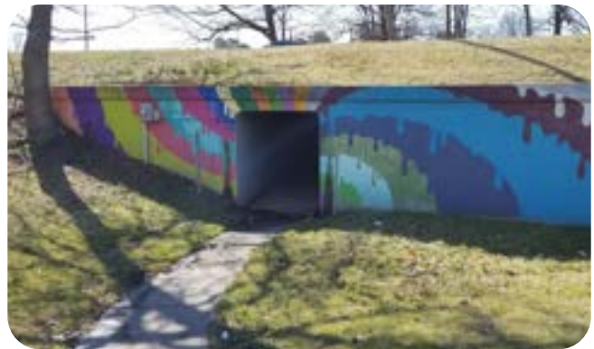
▲ Pedestrian tunnel under Gate City Boulevard
