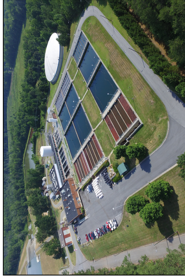
Townsend Water Treatment Plant
