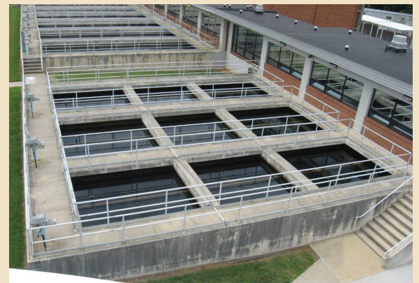
Lake Townsend Water Treatment Plant Filter Basins
