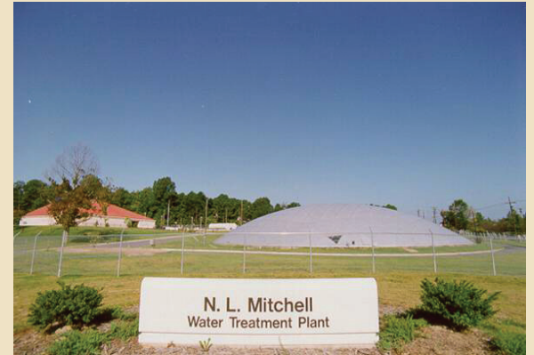
Mitchell Water Treatment Plant Finished Water Reservoir
