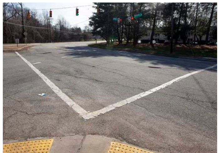
Well-marked, highly visible pedestrian crossings make people feel safer when walking. Pictured above: Fleming at Old Oak Ridge Road.
