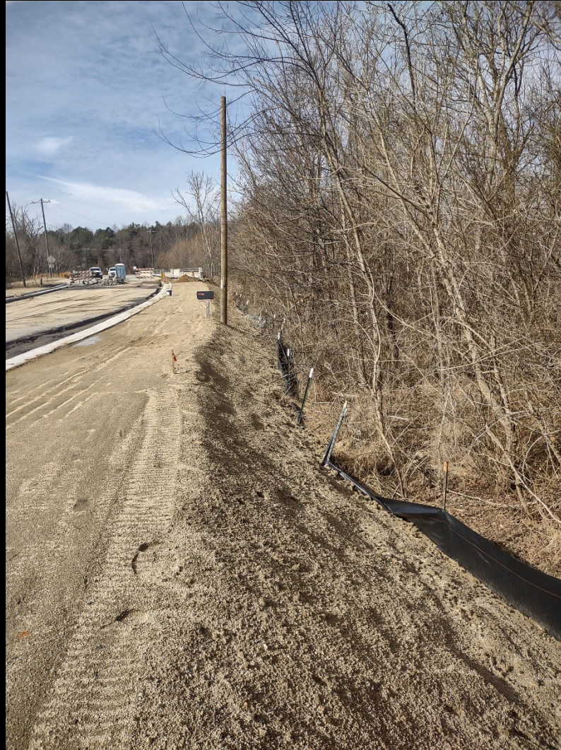
Ballinger Road Bridge
