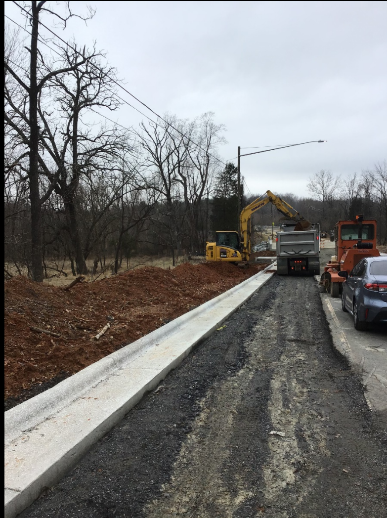
Ballinger Road Bridge
