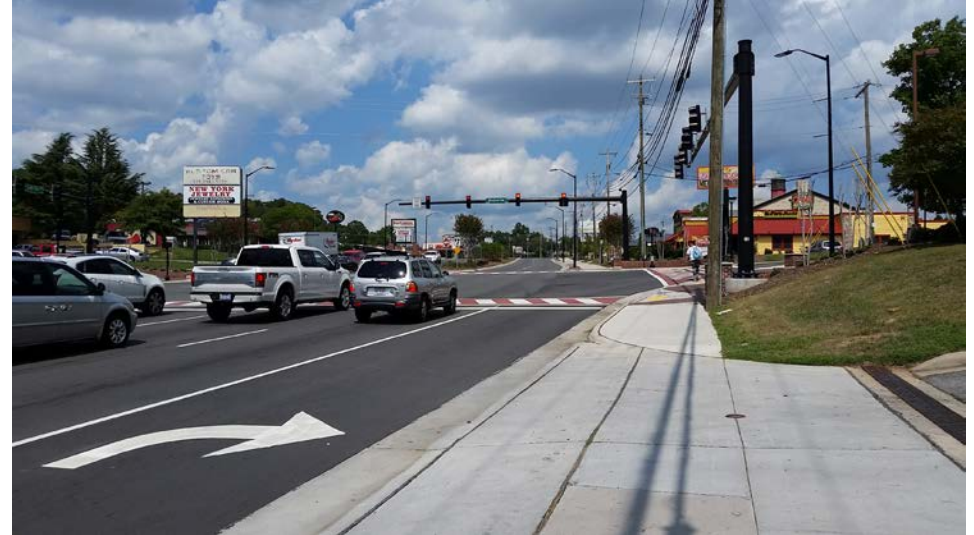
West Gate City Boulevard, after streetscape improvements
