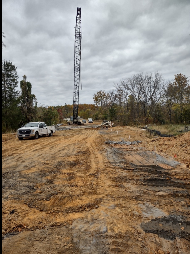
Ballinger Road Bridge
