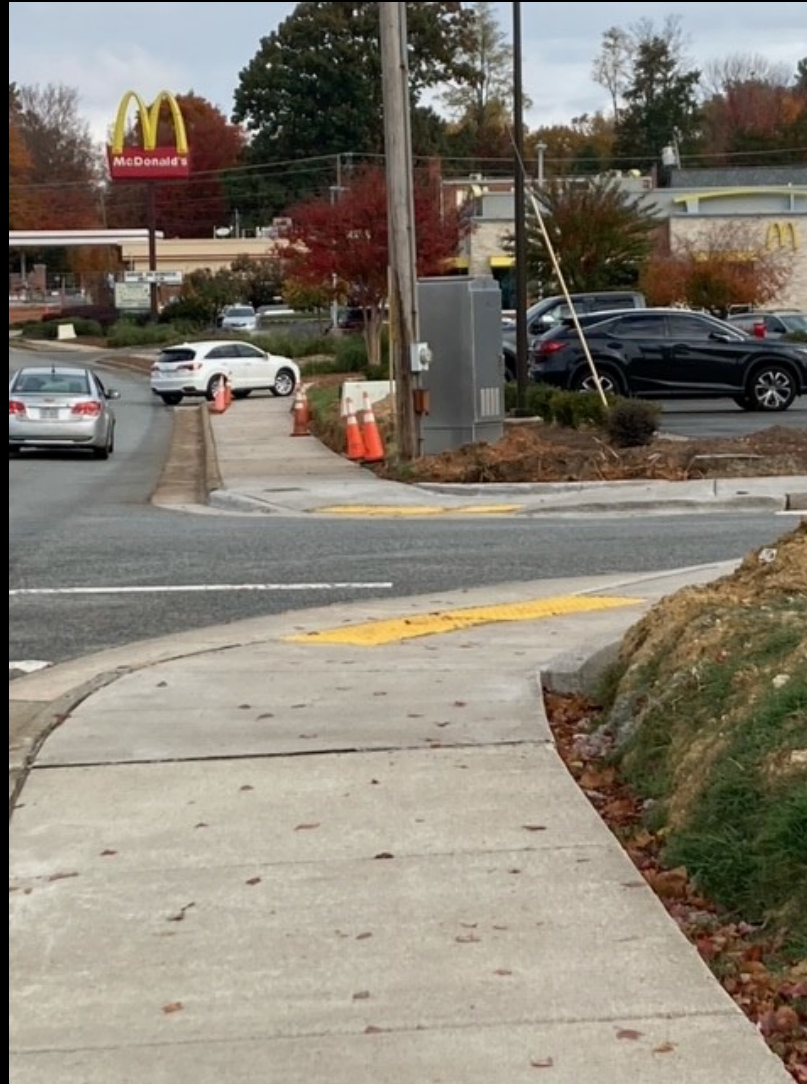
College Road Sidewalk
