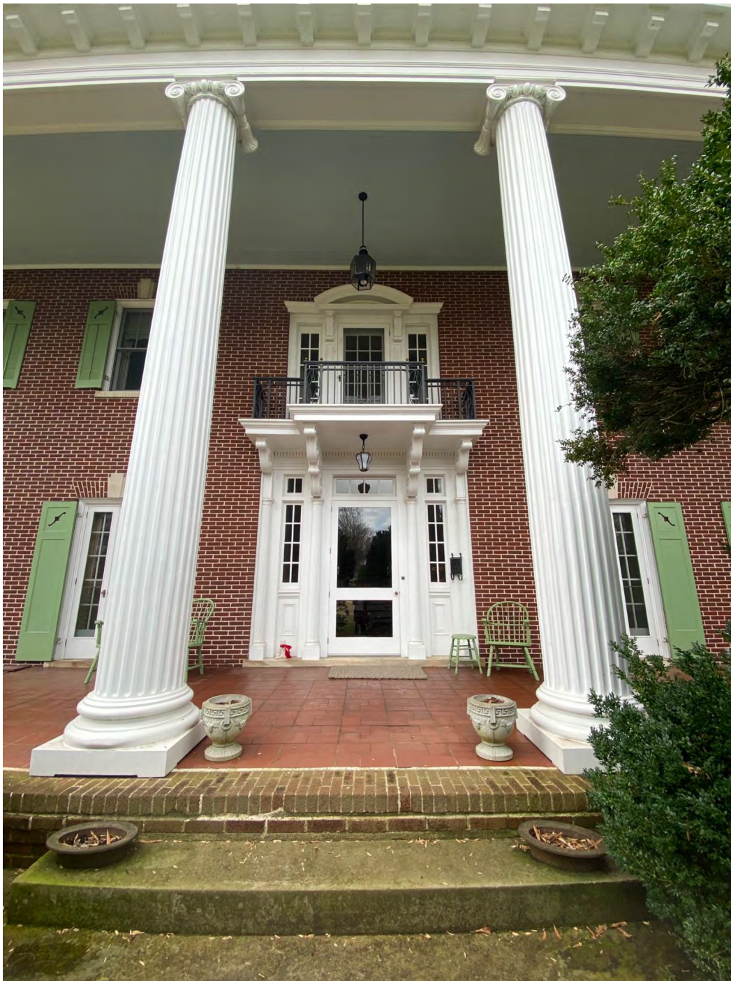
Photo 7a: Facade (north) elevation ionic columns.
