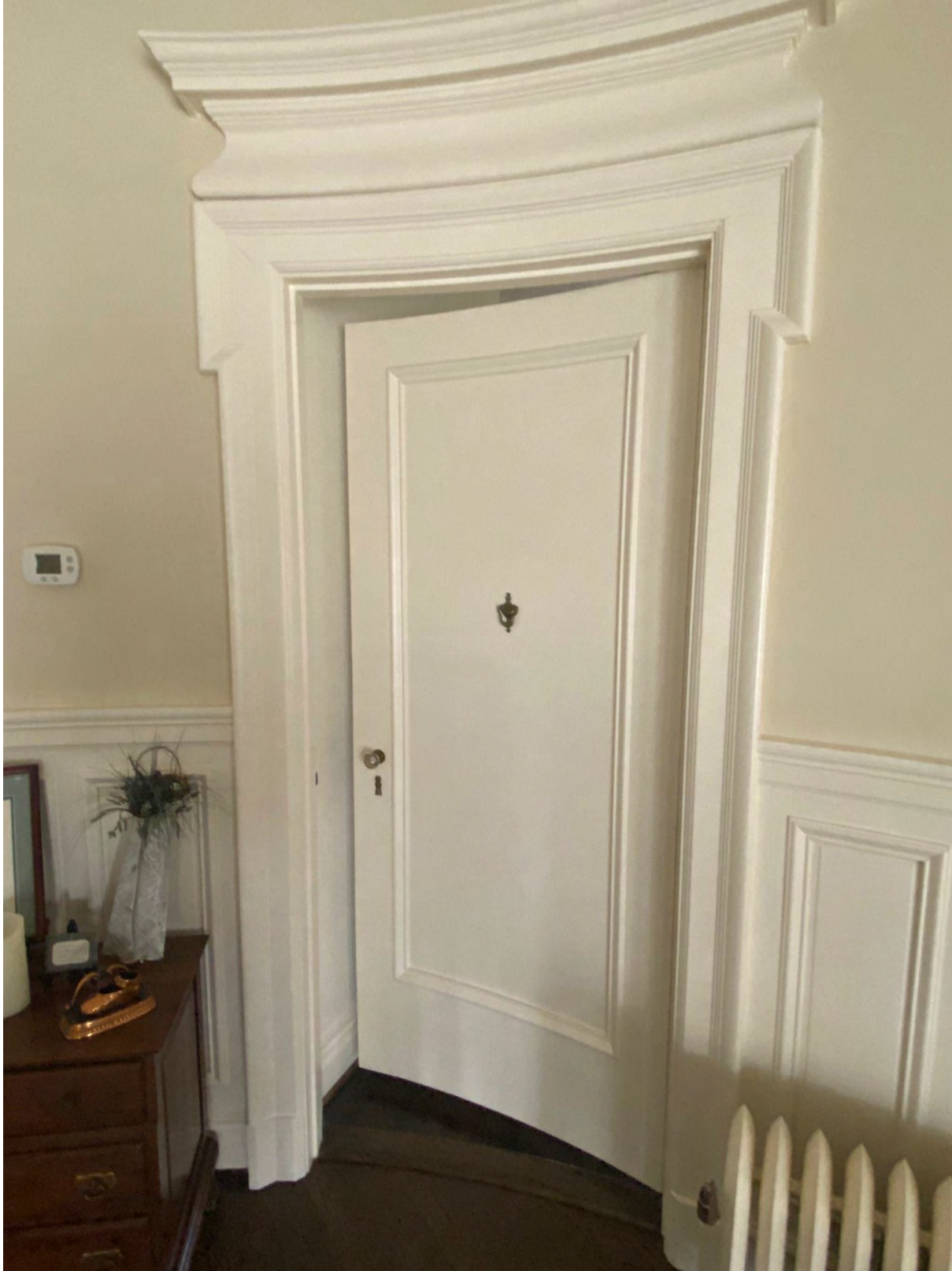
Photo 11n: Curvilinear bedroom door on second level landing
