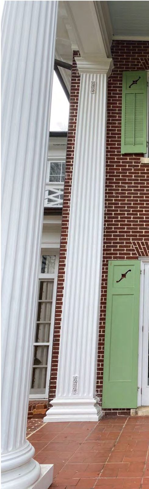
Photo 8: Inset pilaster on the north elevation
