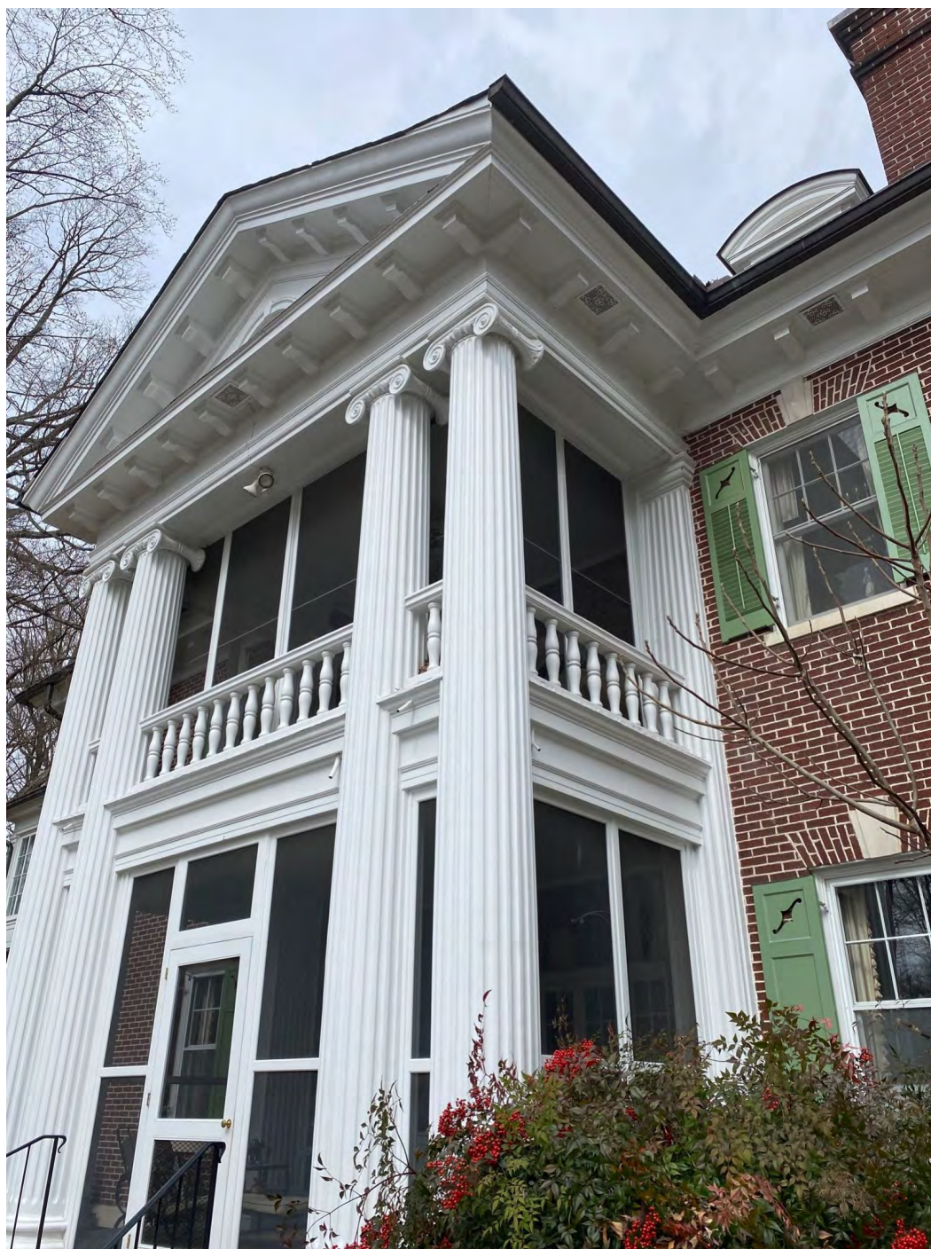
Photo 7b: Rear (south) elevation ionic columns and pedimented portico
