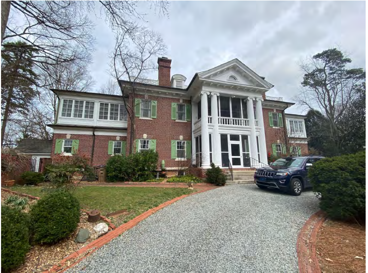
Photo 5: Rear (South) Elevation
