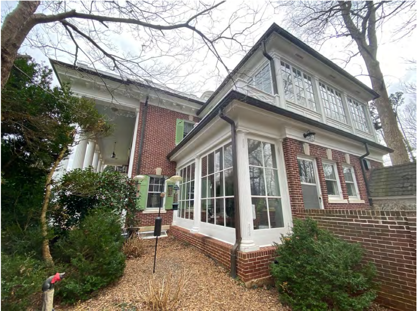
Photo 4: Side (West) Elevation
