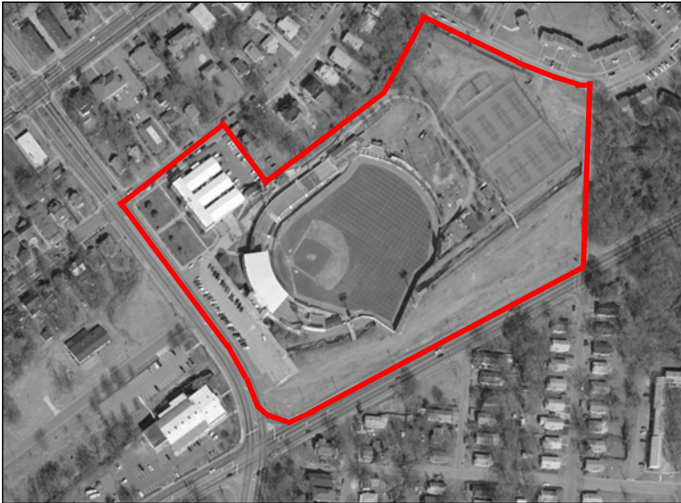
Memorial Stadium site—aerial view of existing block and adjacent site conditions
