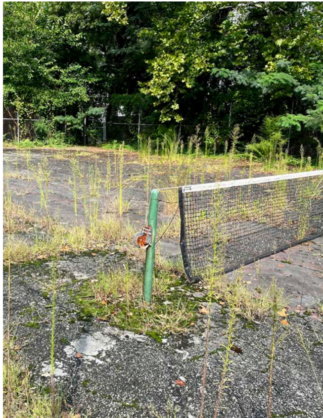
Figure 13 - Existing tennis court.
