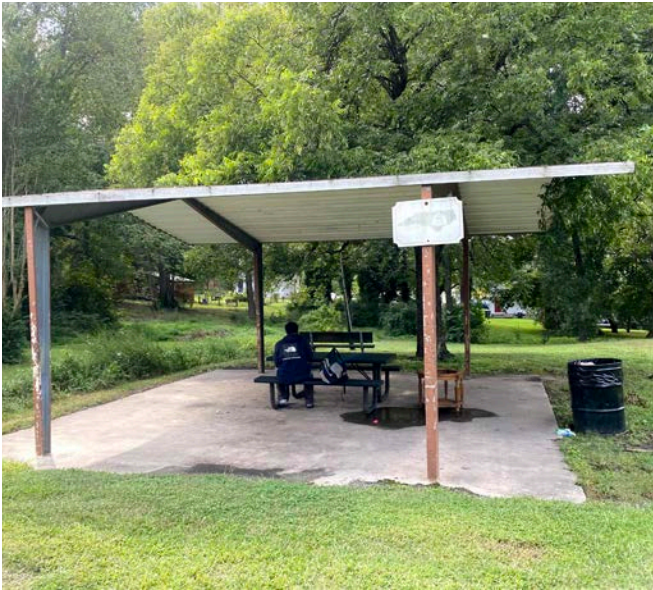
Figure 11 - Existing picnic shelter.
