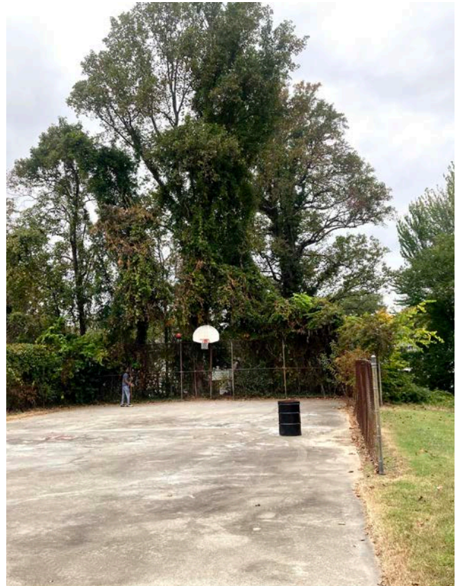
Figure 14 - Existing basketball courts.
