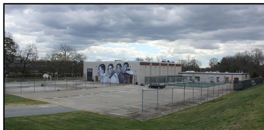
Figures 101 and 102: Windsor Community Center, 1601 East Gate city Boulevard (GF9134)
