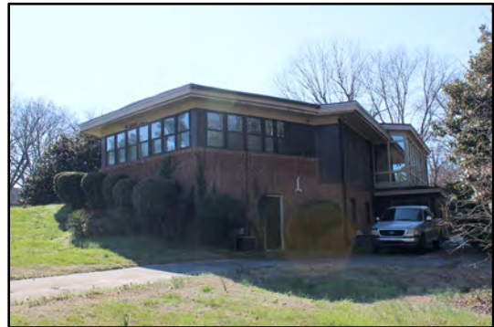
Figures 62 and 63: J. Kenneth Lee House (GF6168) 1021 Broad Street, facing north (top) and west (bottom)
