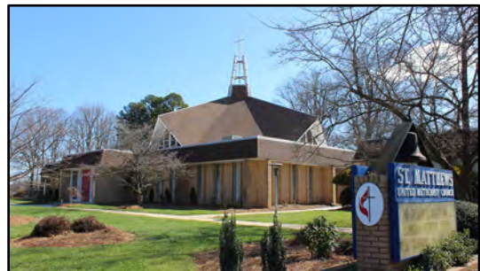
Figure 33: Saint Matthews United Methodist Church (GF9131) 600 East Florida Street
