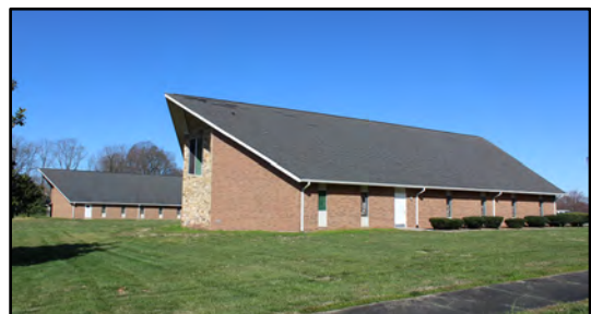
Figure 34: Saint Stephen United Church of Christ (GF9136) 1000 Gorrell Street
