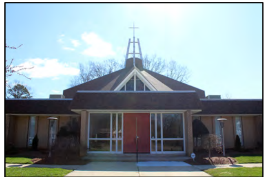
Figure 36: Saint Matthews United Methodist Church (GF9131) 600 East Florida Street
