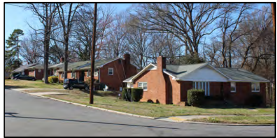
Figure 47: 1200 block Julian Street
