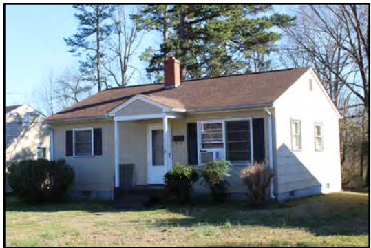
Figure 18: Claude Patterson House (GF6071) 1112 Stephen Street
