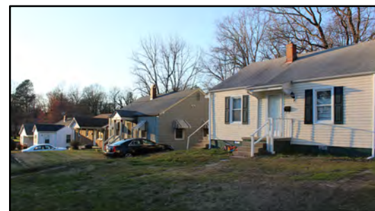
Figure 45: 1400 block Julian Street
