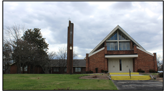
Figure 2: St. James Presbyterian Church (GF2037) 820 Ross Avenue
