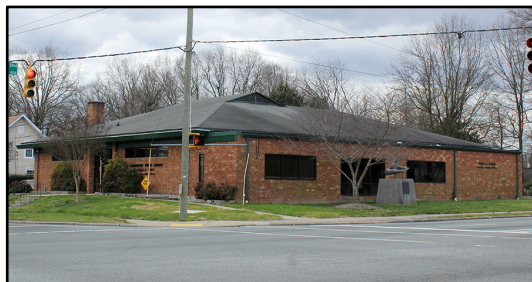
Figure 6: Vance Chavis Library (GF9127) 900 South Benbow Road
