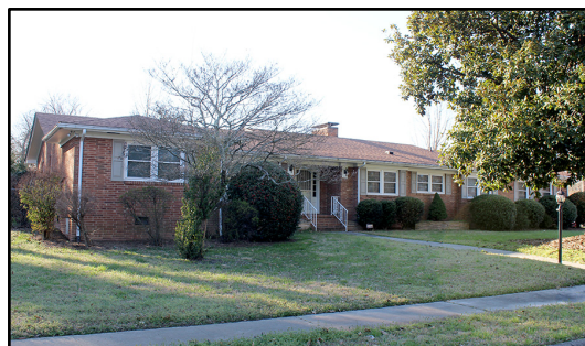
Figure 10: 1500 Marboro Drive (GF9144)
