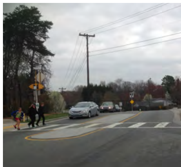
Crossing improvements at trail and greenway crossings require several elements, including signals, signs, high-visibility crosswalks and medians.
