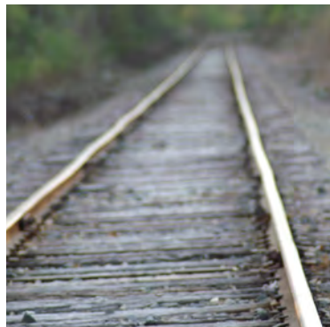
The construction of the A&Y Greenway will add two miles to the greenway system in the City.
