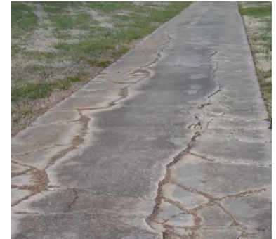
Deteriorating pavement is a long-term maintenance concern for all greenways that must be addressed.
