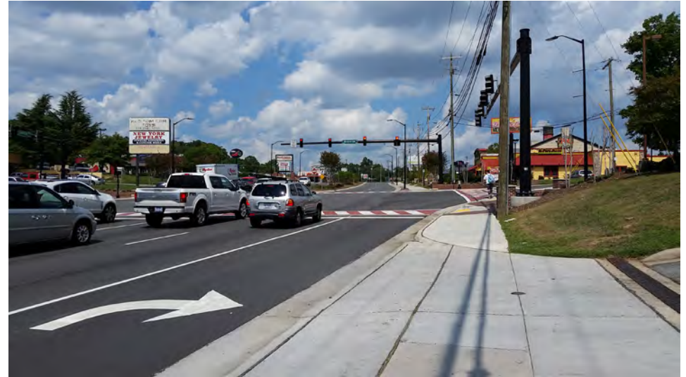
West Gate City Boulevard, after streetscape improvements
