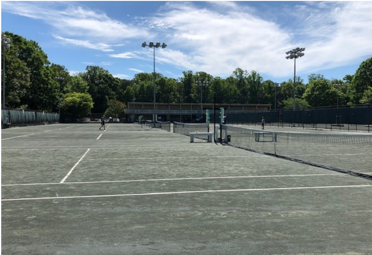
Renovated Clay Courts at Spencer Love Tennis Center (Phase 1)
