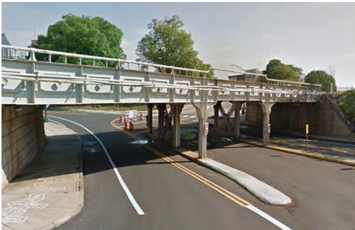
Existing condition along East McGee Street
