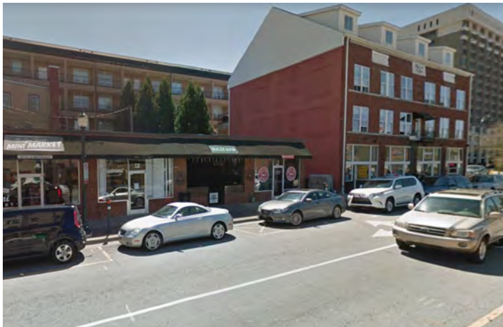
Existing condition along West McGee Street
