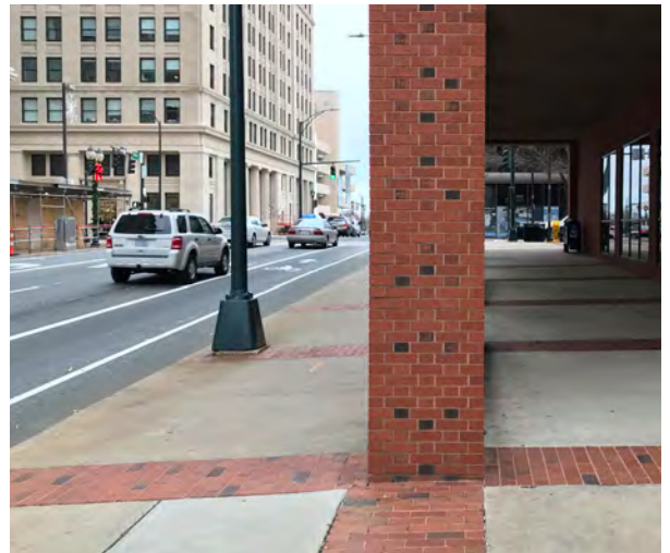
Existing condition along Market Street
