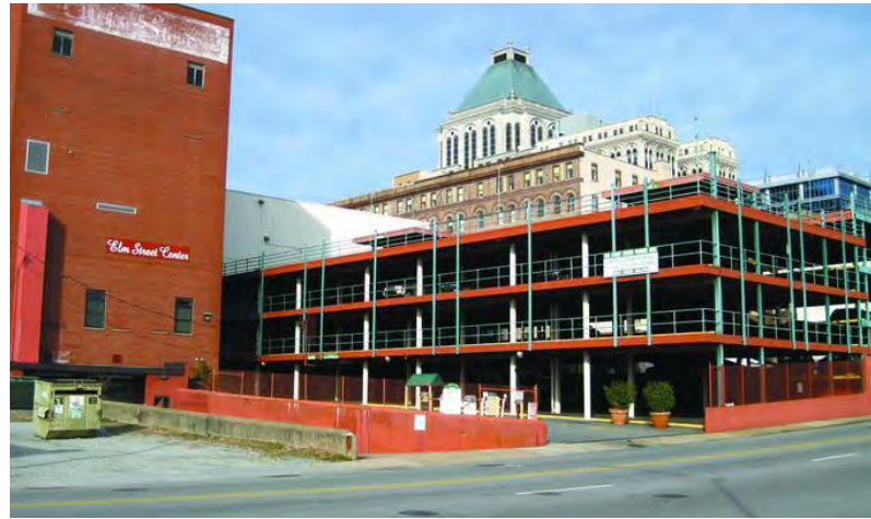
Site for future development along Davie Street
