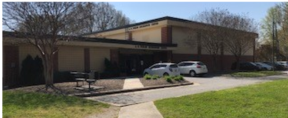
Existing Conditions — Peeler Recreation Center
