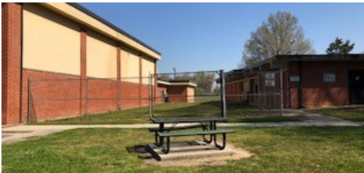
Underutilized Area at Rear of Recreation Center
