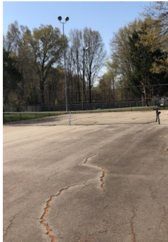
Existing Conditions – Tennis Courts
