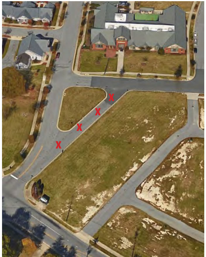
Gateway entry roundabout and red X's displaying partial elimination of Lincoln Street. and spur between McConnell Road and Everitt Street
