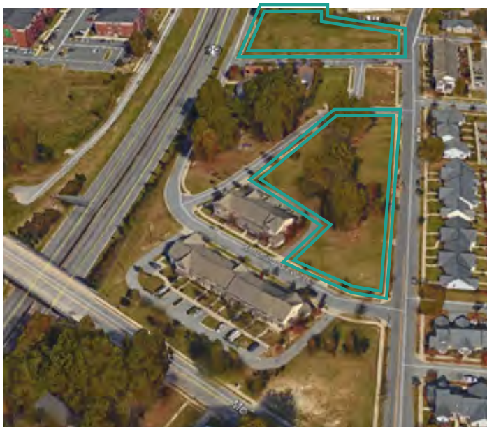
Figure 30: Northern and southern vacant areas in D1
