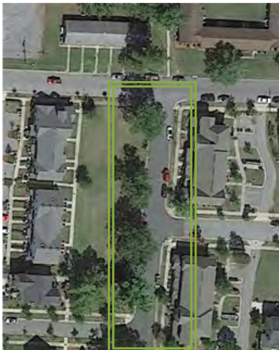
Existing conditions on Jennifer Street between Evans and Spencer
