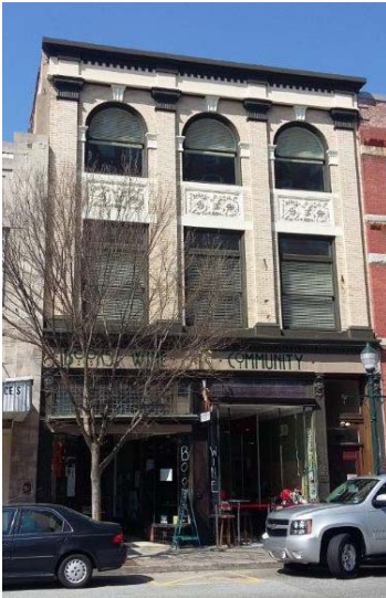
Left: 304 S. Elm Street in the downtown district was restored utilizing tax credits.
