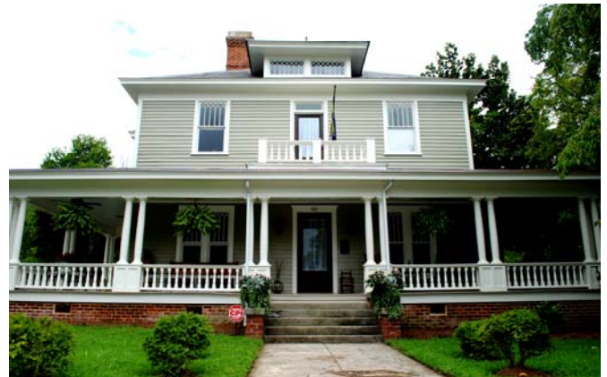
The William A. Crawford House at 919 Spring Garden Street suffered a disastrous fire in 2011. The Planning Department partnered with Preservation Greensboro, Inc and the College Hill Neighborhood Association to save the house from demolition.
