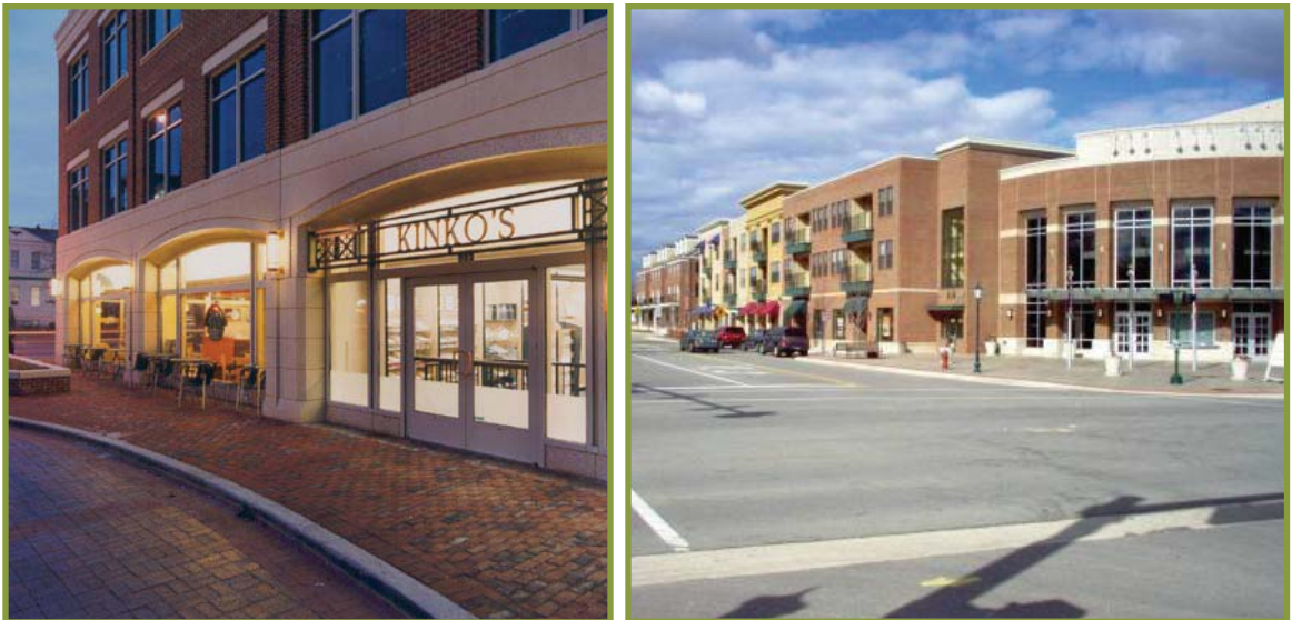
Character examples of ground floor, mixed-use retail with residential housing above.
