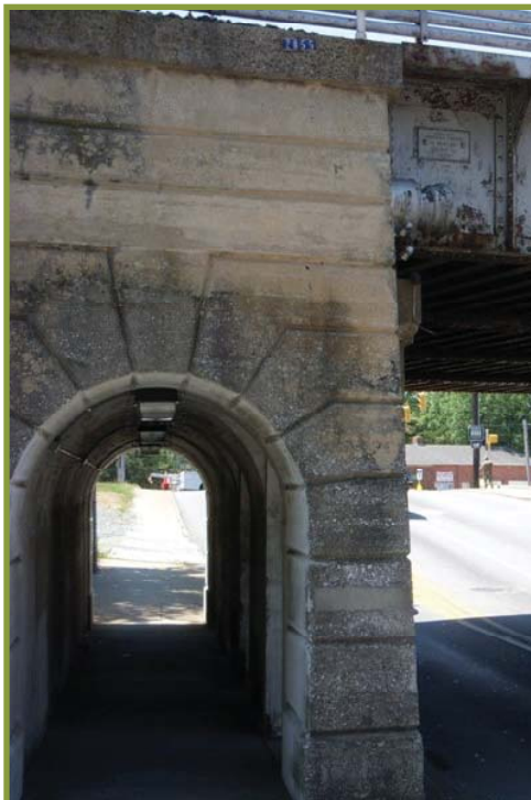
Figure E: Underpass below N.C. Railroad
