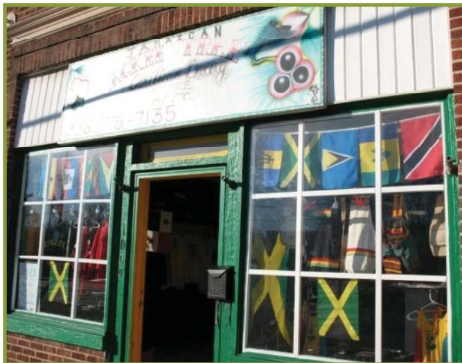
Existing Building Facade
