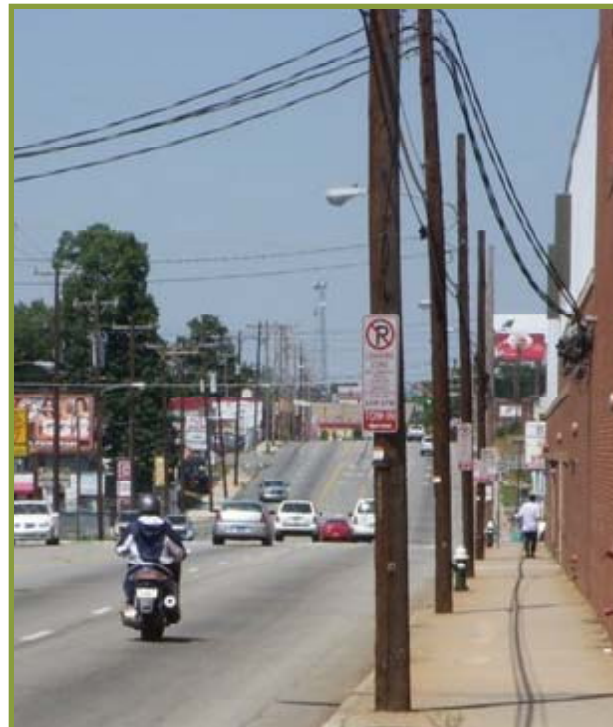
Figure F: Utility poles obstructing sidewalk
