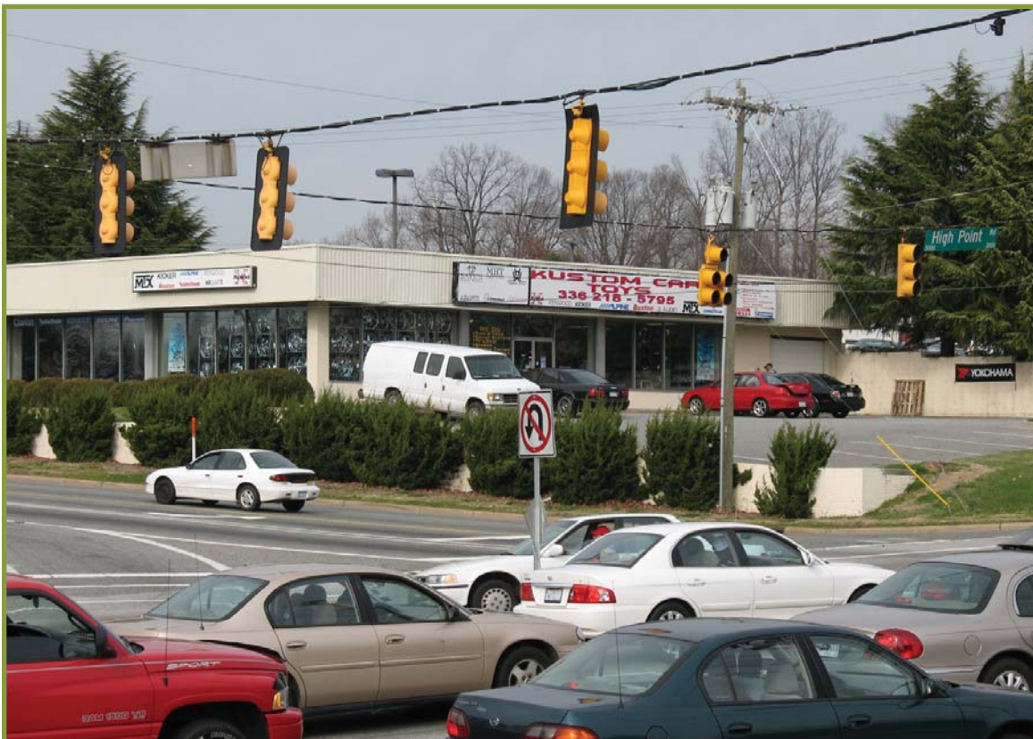
Existing traffic signals strung between utility poles
