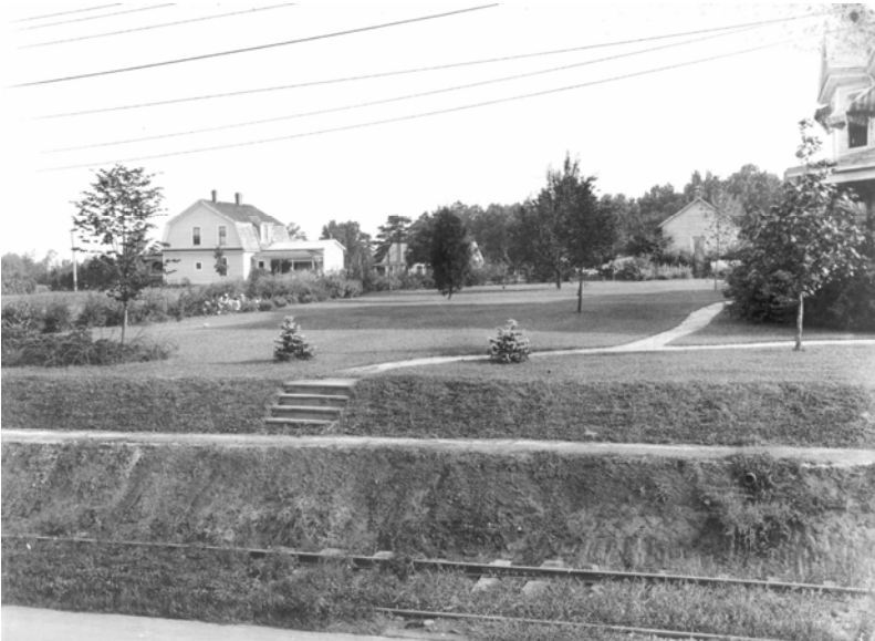
Residences Located Near a Street Car Line
